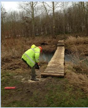
At the AGM last November a member notified the BAA that the footbridge over the stream at Wick was in a poor state and required repair. The rotten timber supports and planks have now been replaced with new. The photo above shows the footbridge after repair.
