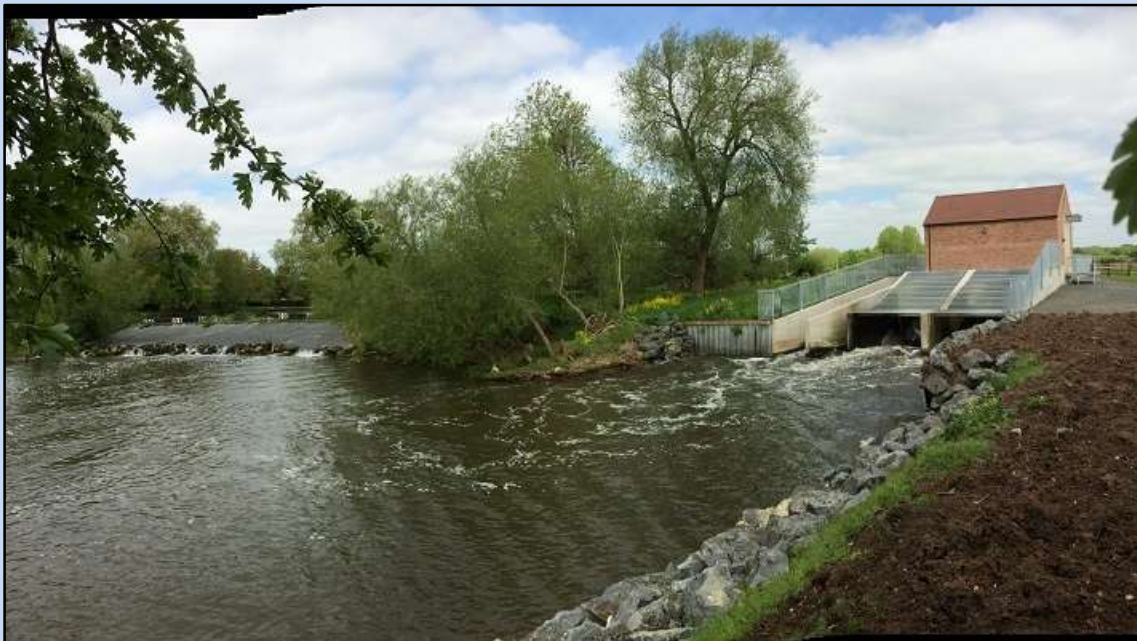
Hydro plant alongside Pershore weir
