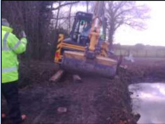
Getting JCB onto bank to fix leak
