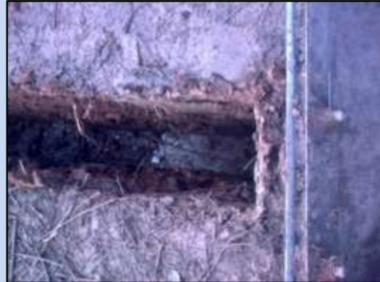
Leak dug out and ready to be filled.
